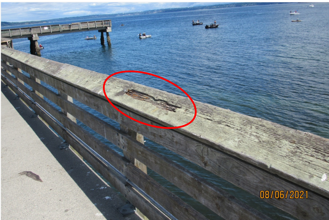
Photograph 22 – View of decay in the east top railing board, near Bent 3.4 shown, looking northeast
