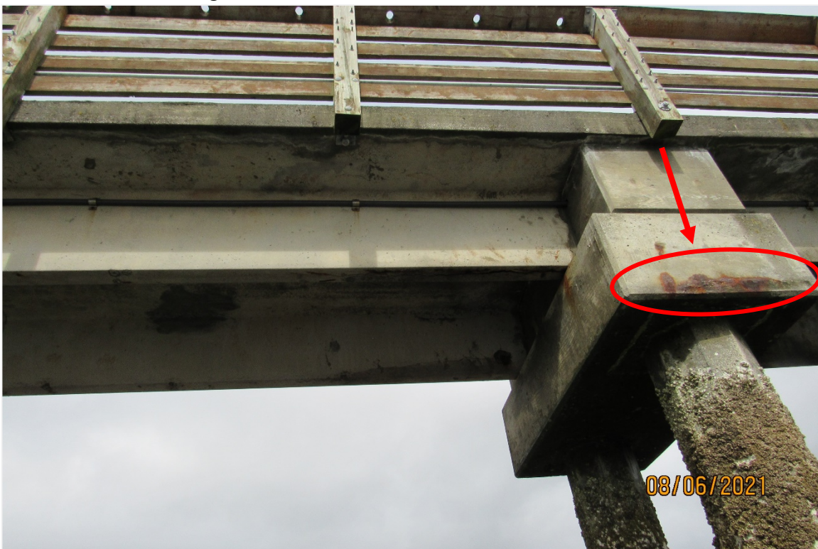
Photograph 6 – View of the rust staining typical condition, Bent 3 pile cap shown, looking west
