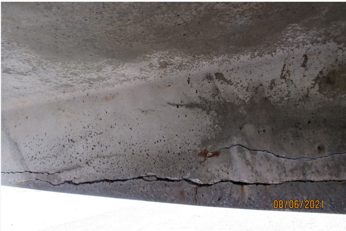
Photograph 8 – View of a typical closed corrosion spall, near Bent 1 shown, looking east
