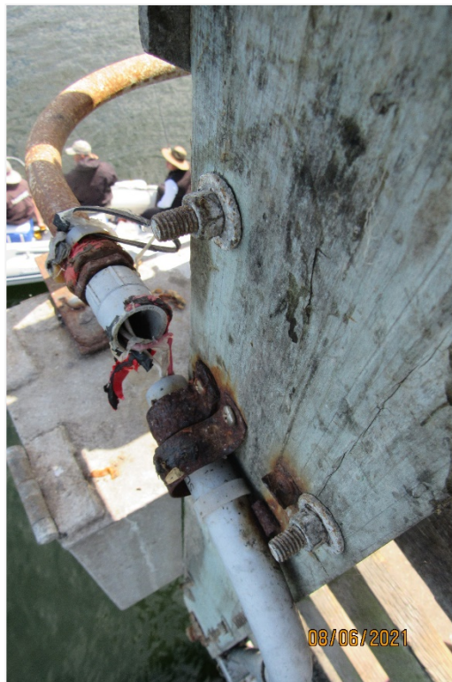
Photograph 26 – View of the disconnected navigational utility line at Bent 10, looking east
