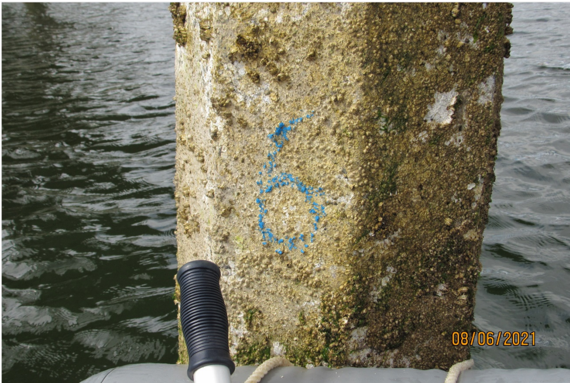
Photograph 3 – View of marine growth on the precast prestressed concrete pile, Pile 6;B shown, looking southwest
