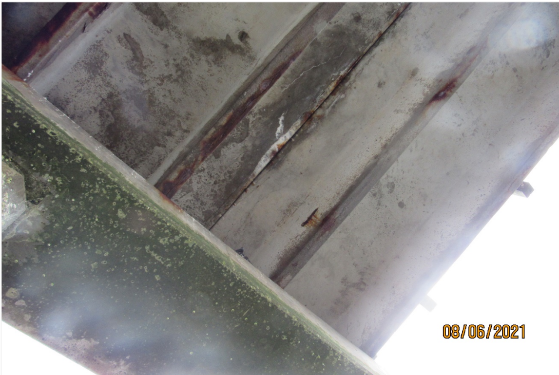
Photograph 15 – View of delamination and staining in the beam top flange, near Bent 8 shown, looking northwest
