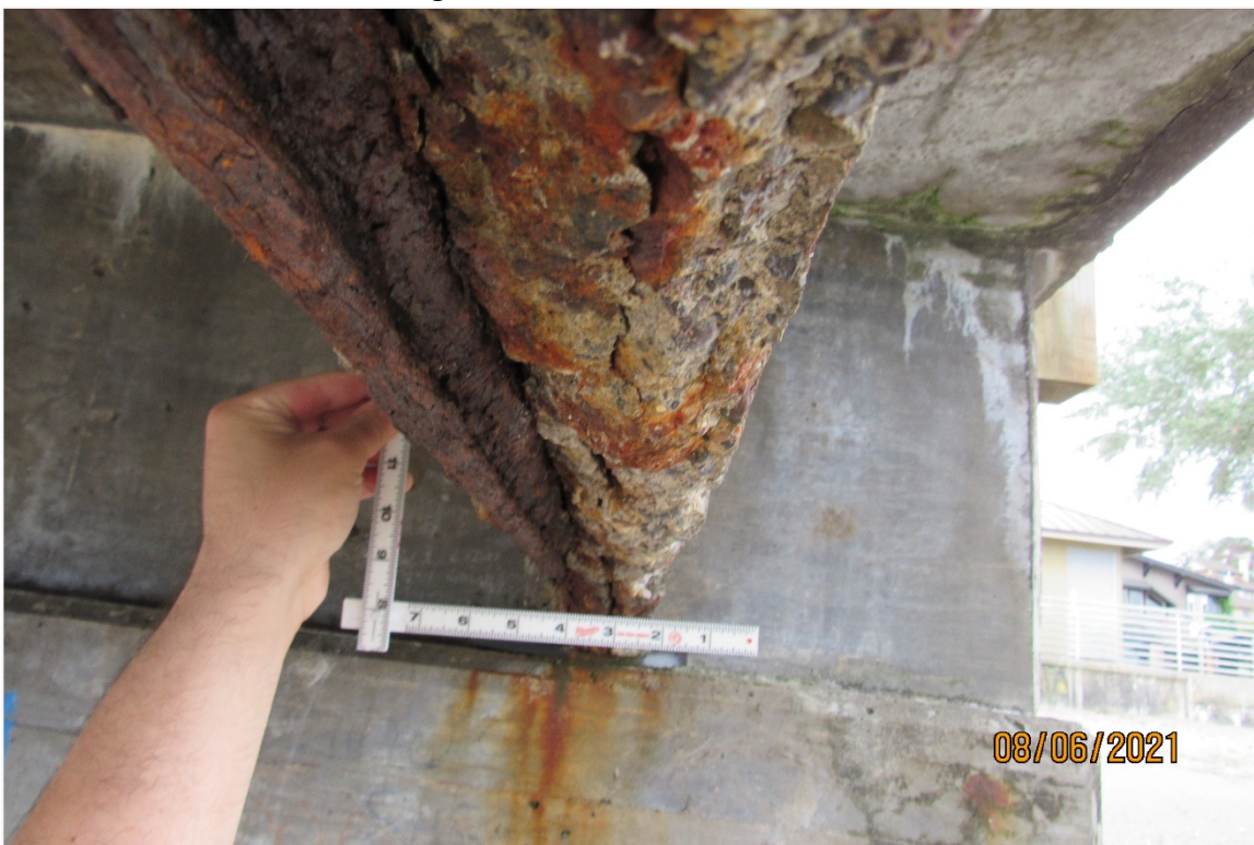
Photograph 10 – View of an open corrosion spall with exposed steel, near Bent 1 shown, looking south
