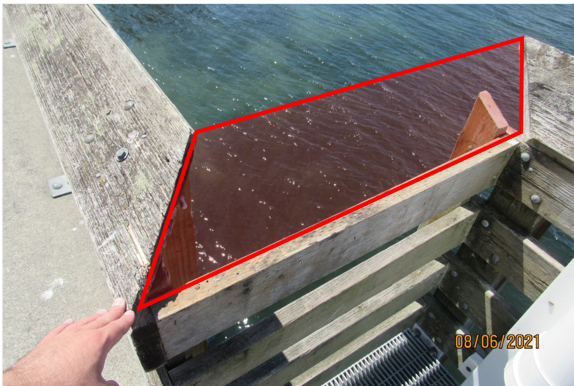
Photograph 24 – View of the west missing top railing at Bent 4, looking southwest
