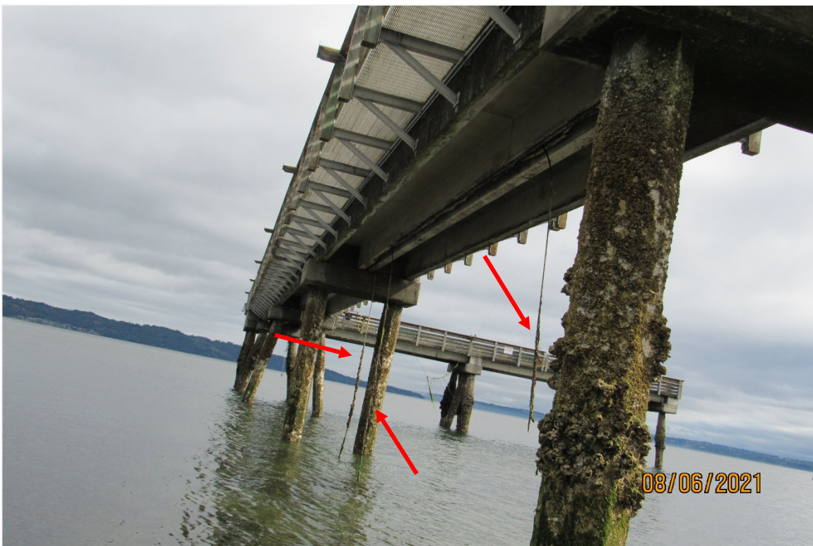
Photograph 12 – View of an open corrosion spall and three broken prestressing strands, Bent 4.5 shown, looking north
