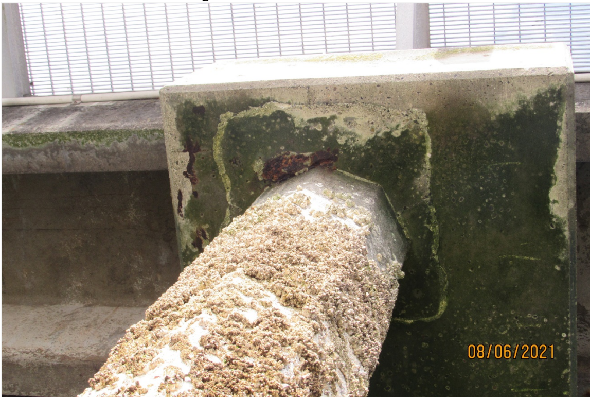
Photograph 4 – View of the typical concrete pile condition, Pile 5;B shown, looking west
