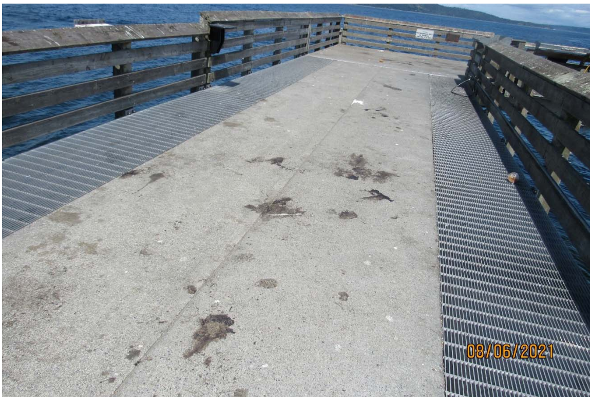
Figure 3.2.4-1. View of typical concrete topping slab and aluminum grating condition, near Bent 6, looking north.
