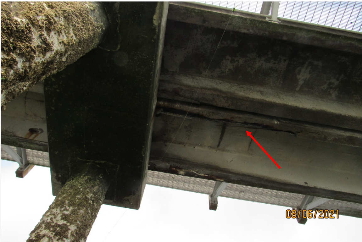
Photograph 13 – View of an open corrosion spall with two broken prestressing strands, Bent 5.2 shown, looking west
