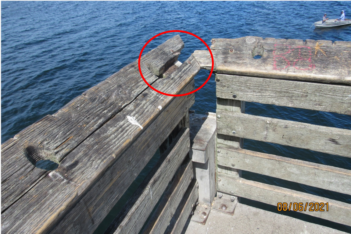
Photograph 25 – View of the broken top rail at the northwest corner of Bent 8, looking north
