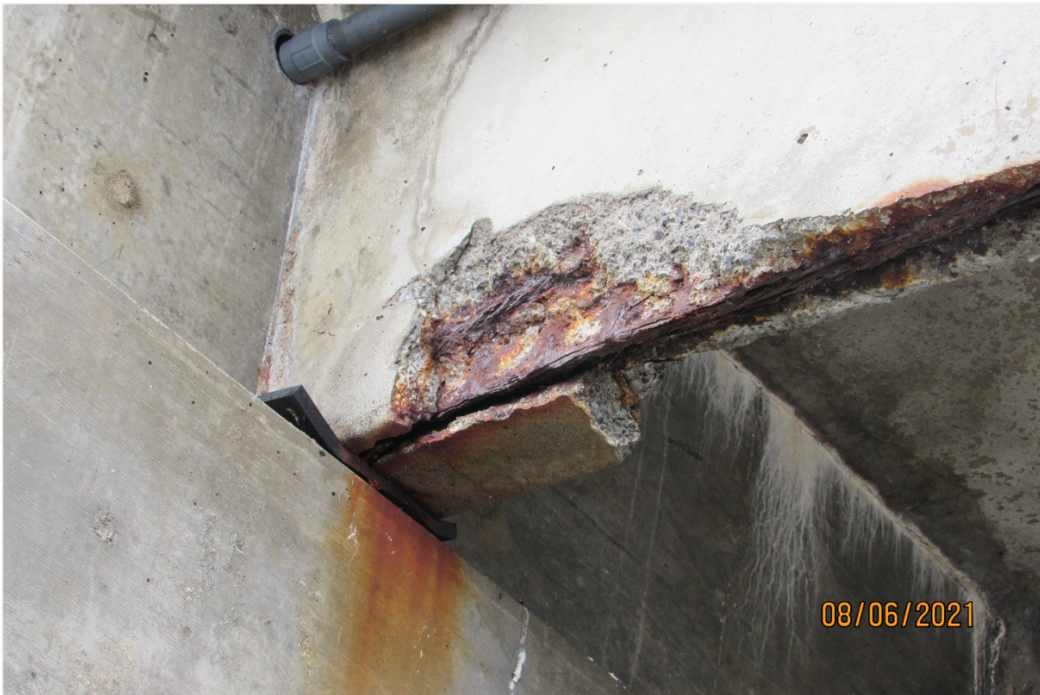
Photograph 11 – View of an open corrosion spall at the bearing, Bent 2N shown, looking southwest
