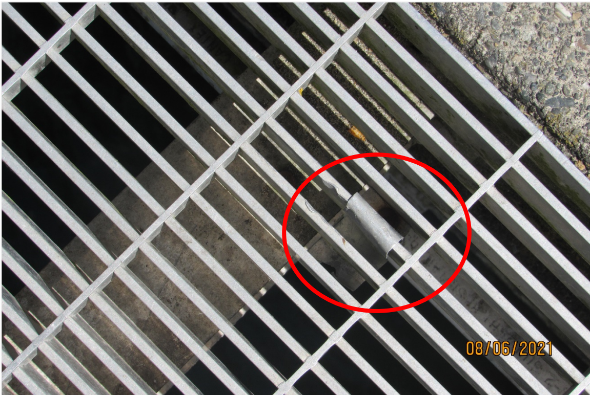
Photograph 19 – View of a typical broken clip that secures the aluminum grating, looking north
