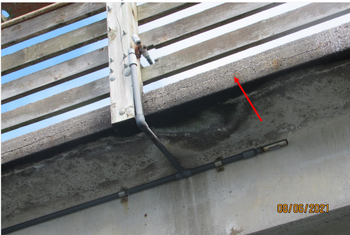
Photograph 16 – View of a longitudinal crack in the beam top flange, near Bent 9 shown, looking north
