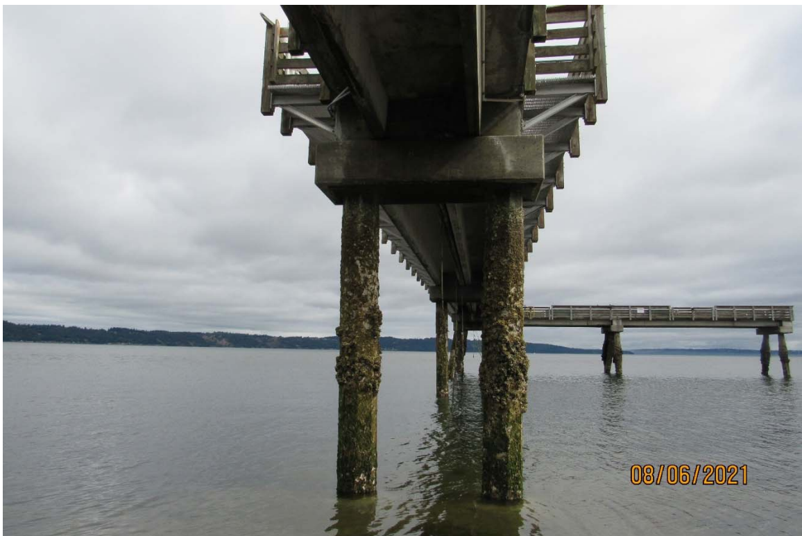
Figure 3.2.1-2. View of typical structural pile configuration, Bent 4 shown, looking North.
