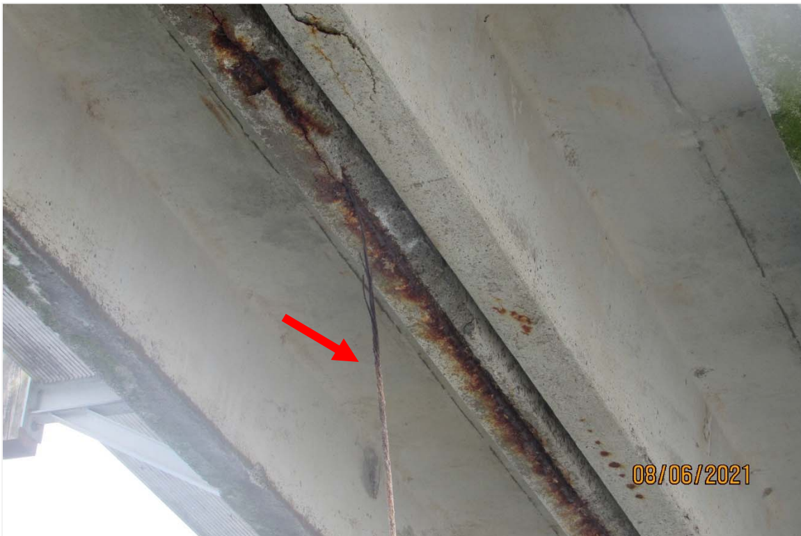
Figure 3.2.3-2. View of severe spalling and broken pre-stressing strand in beam, Bent 6.5 shown, looking north.
