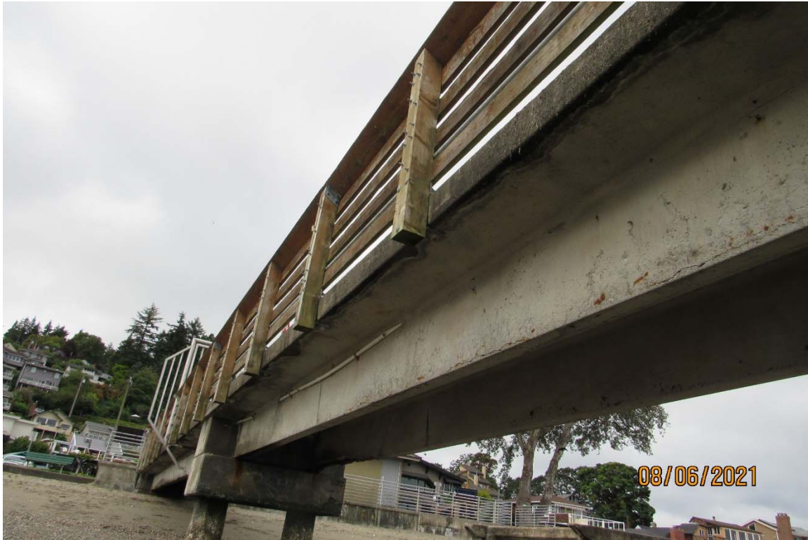
Figure 3.2.3-1. View of typical concrete beam configuration, Span 2 shown, looking south.
