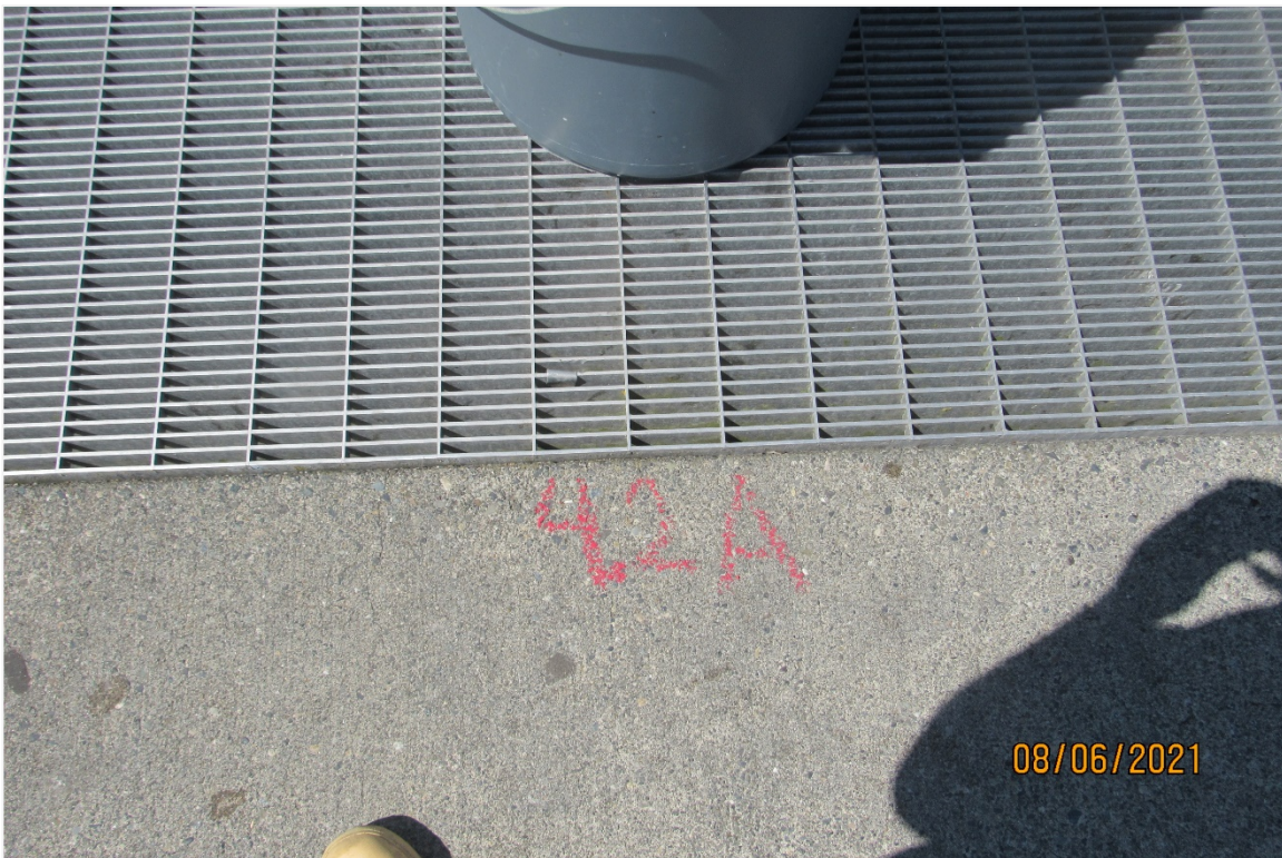
Photograph 18 – View of the typical aluminum grating condition, near Bent 4.2 shown, looking west
