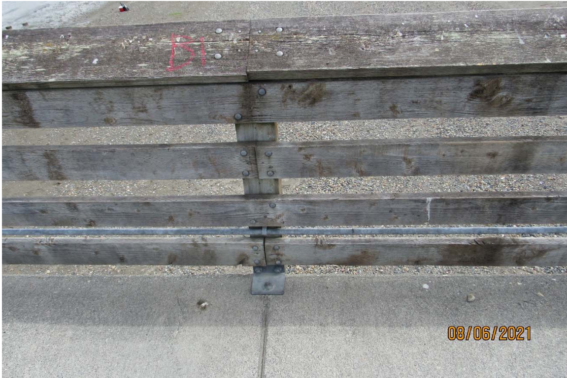
Figure 3.2.5-1. View of the typical timber railing and post condition, near Bent 1 shown, looking east.
