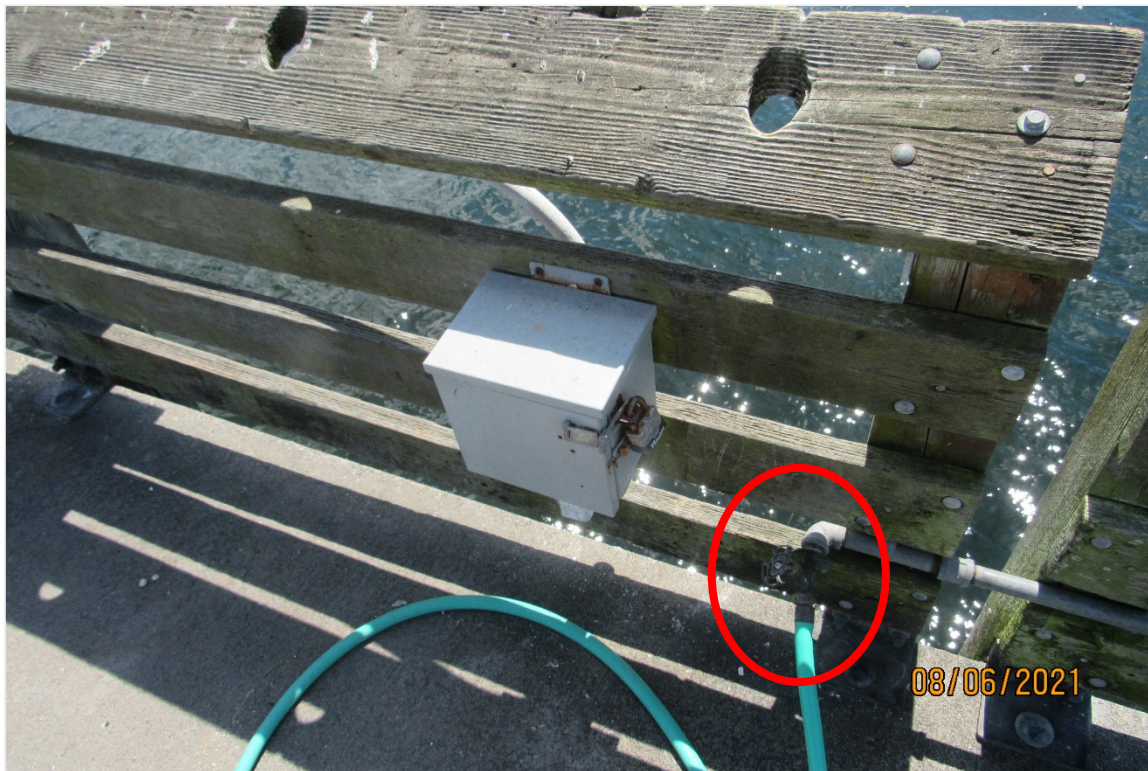
Photograph 28 – View of the potable water receptacle bib at Bent 8.5, looking south
