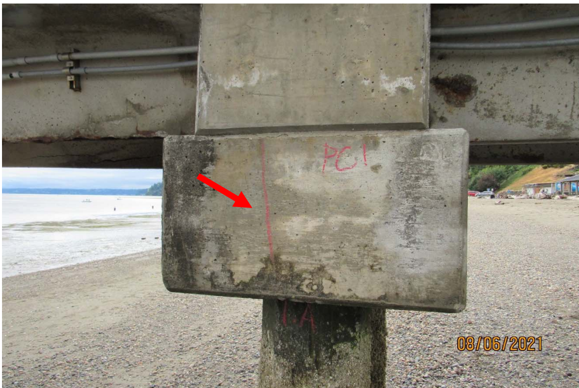
Figure 3.2.2-2. View of vertical cracking in the west face of the Bent 1 pile cap, looking east.
