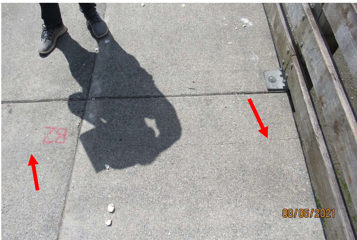
Figure 3.2.4-2. View of transverse cracking in the top slab at Bent 2, looking south.
