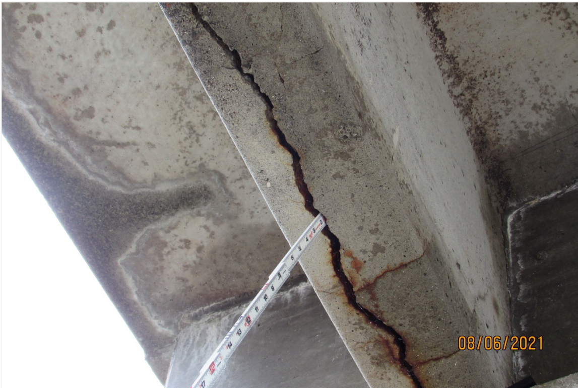
Photograph 9 – View of a typical crack in the bottom face of the beam web, near Bent 2 shown, looking south
