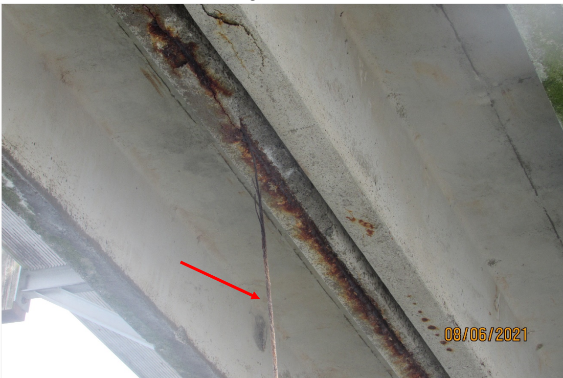
Photograph 14 – View of an open corrosion spall with a broken prestressing strand, Bent 6.8 shown, looking north
