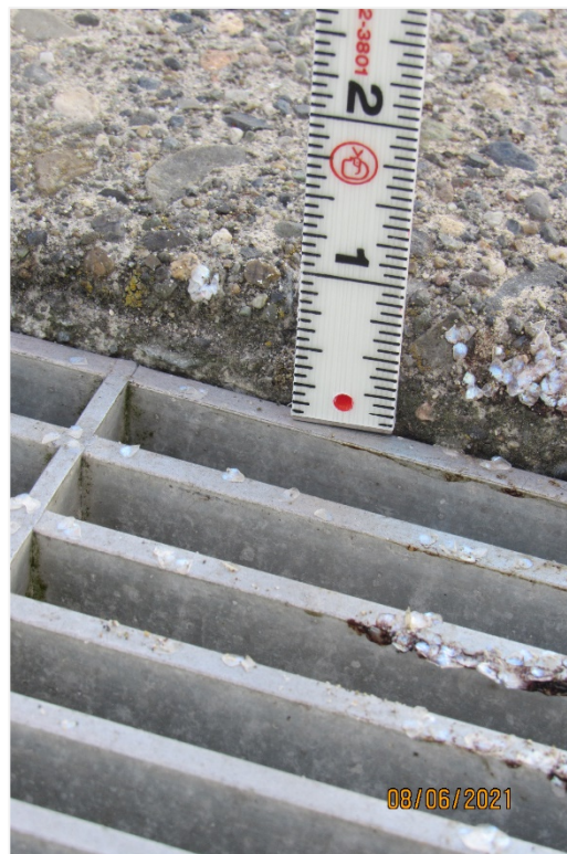
Photograph 20 – View of the misalignment of the aluminum grating and the concrete topping slab, looking east
