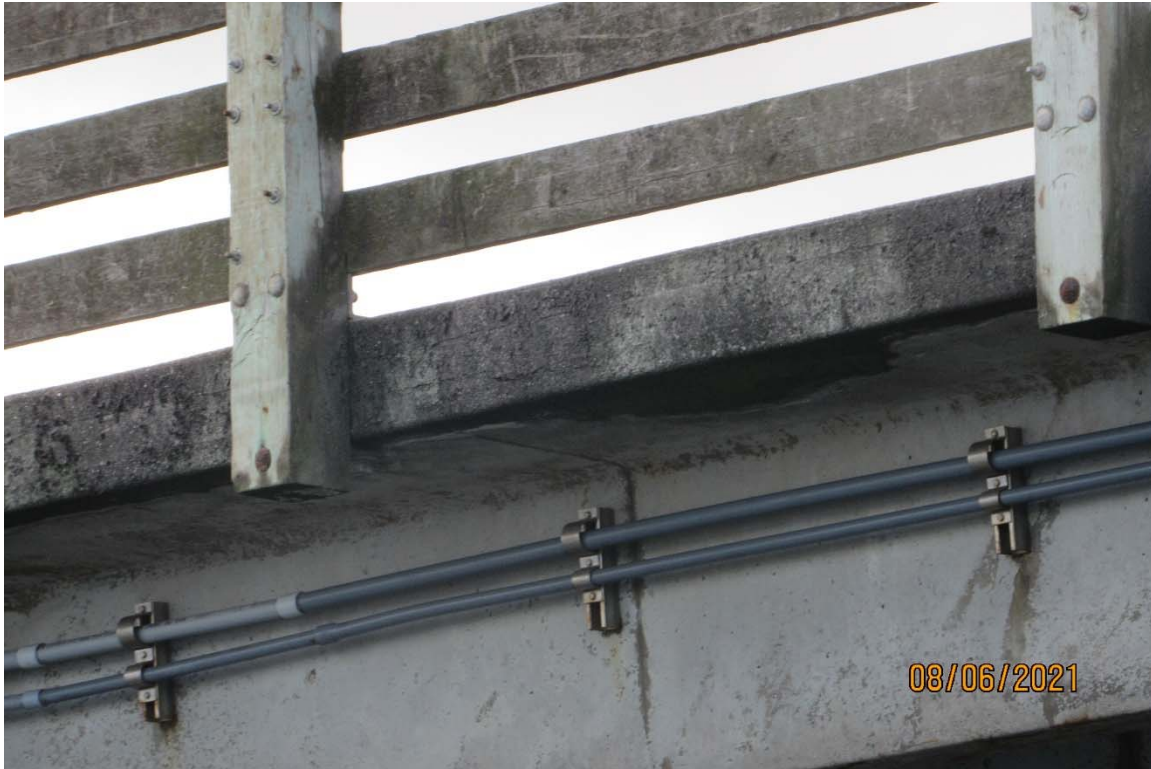
Figure 3.2.5-2. View of the electrical (upper) and navigational (lower) utility line typical condition, looking northeast.
