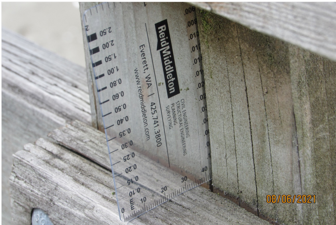
Photograph 23 – View of typical checking in the timber rail posts, looking southwest
