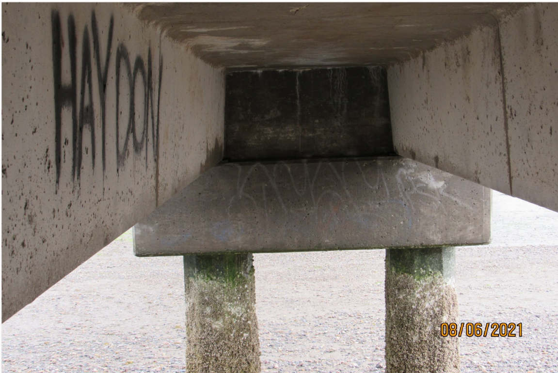
Photograph 5 – View of the typical concrete pile cap condition, Bent 1 pile cap shown, looking north
