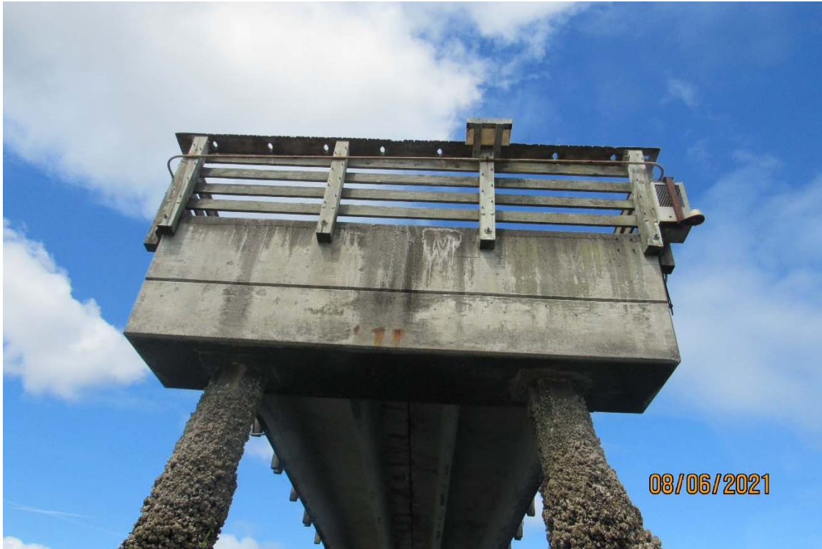
Figure 3.2.2-1. View of the typical pile cap condition, Bent 10 pile cap shown, looking west.
