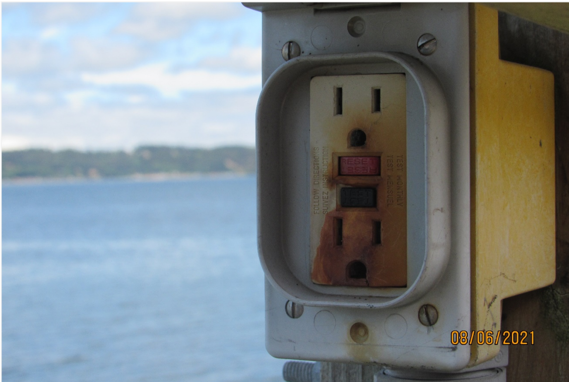
Photograph 27 – View of the typical heavy staining and discoloration on the electrical outlet, looking northwest
